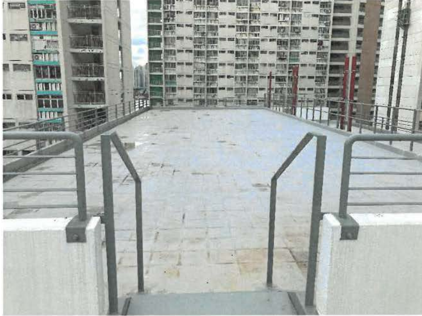
Photo No.: R-1 Location: Roof
