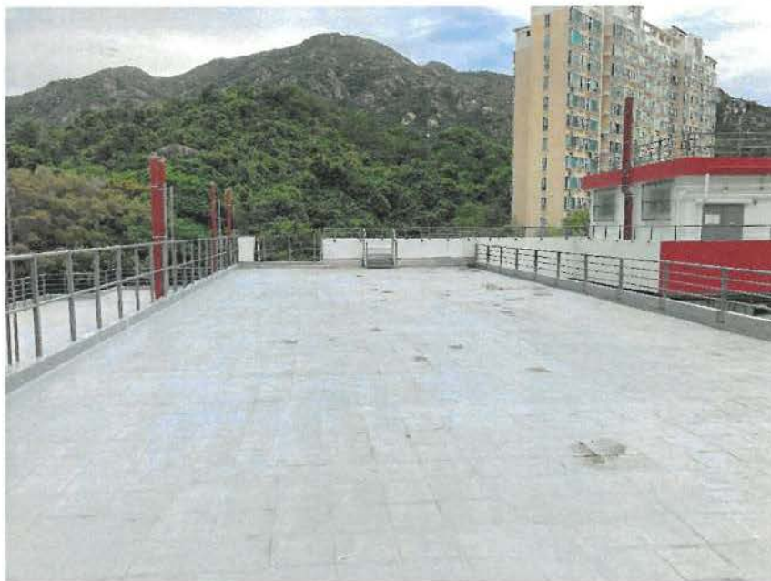
Photo No.: R-2 Location: Roof
