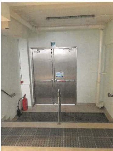
Photo No.: G-16 Location: Exit of Staircase-01 at G/F
