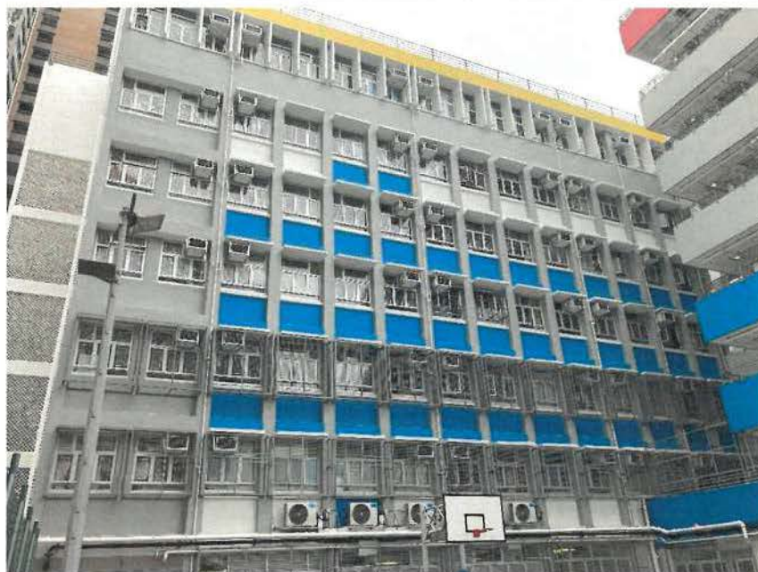
Photo No.: E-3 Location: External wall
