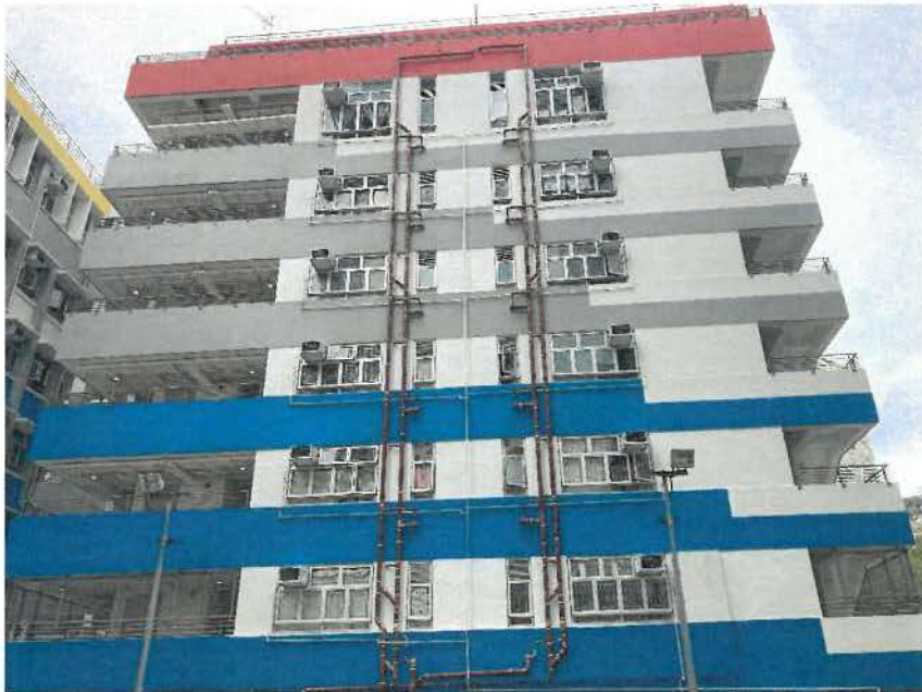
Photo No.: E-2 Location: External wall
