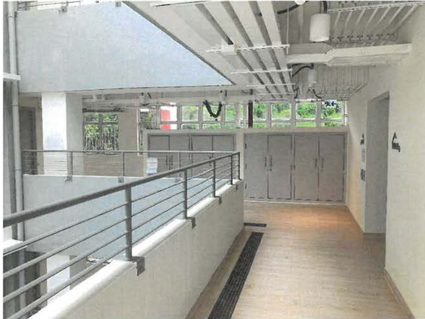
Photo No.: 5-5 Location: Corridor 2 at 5/F
