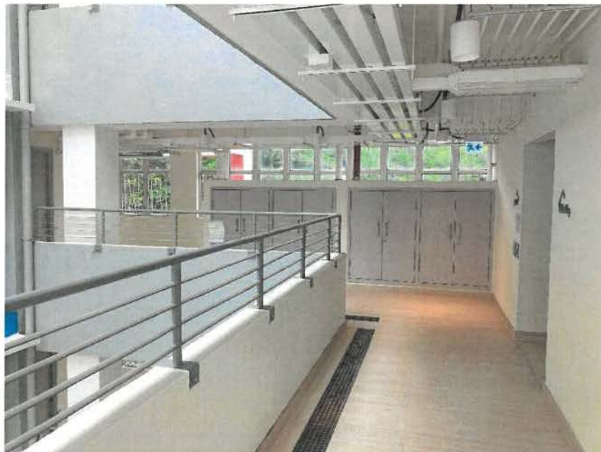
Photo No.: 4-4 Location: Corridor 2 at 4/F
