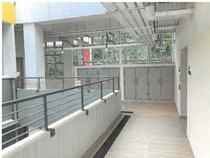
Photo No.: 6-4 Location: Corridor 2 at 6/F
