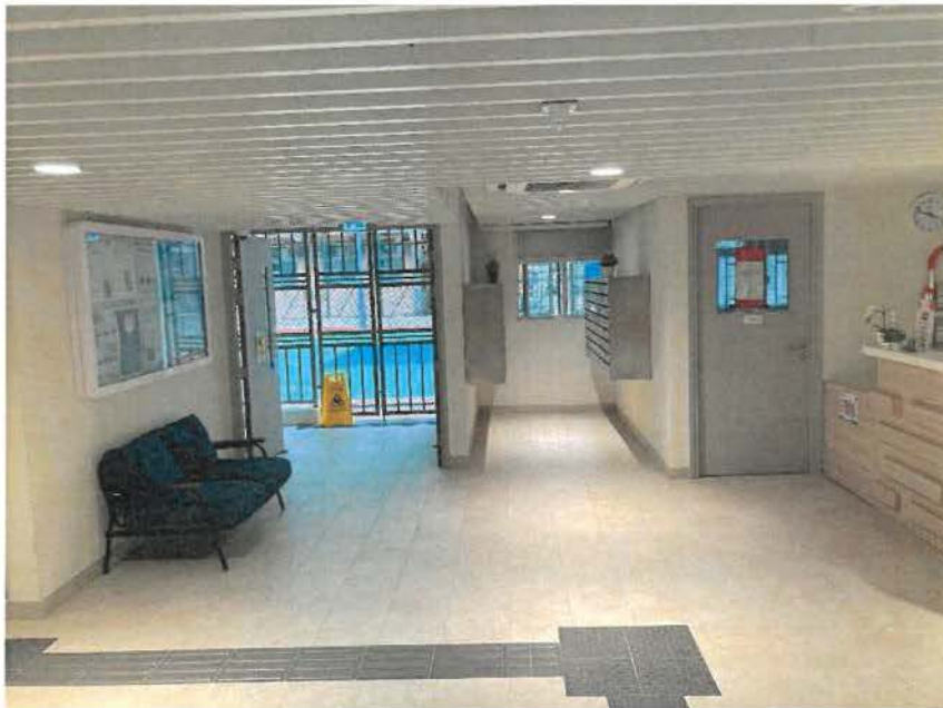
Photo No.: G-2 Location: Reception at G/F
